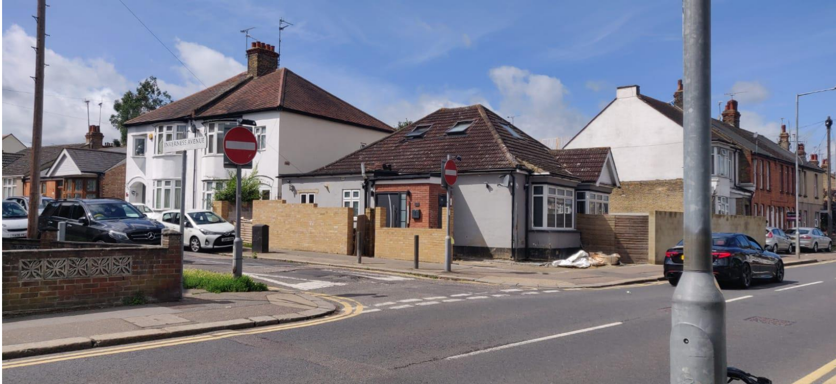
The site from Fairfax Drive showing the new boundary walls, porch and hardstanding
